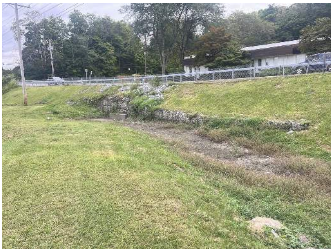
2026 The swallow hole: the channel runs to this limestone seam and the water simply goes down into it. Outdoor Promise, Sept 2026
