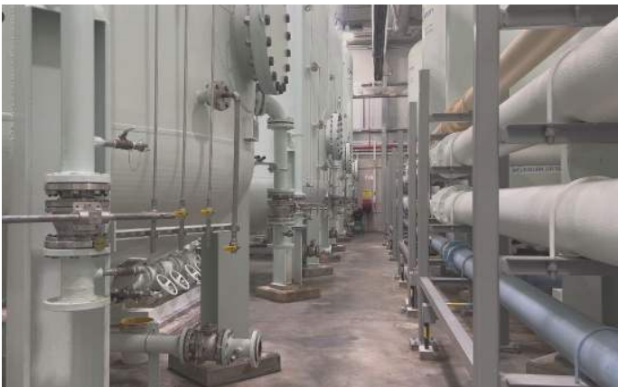
2026 Inside the plant: the big carbon filter tanks the water passes through, and the pipes that feed them. Outdoor Promise, Sept 2026
